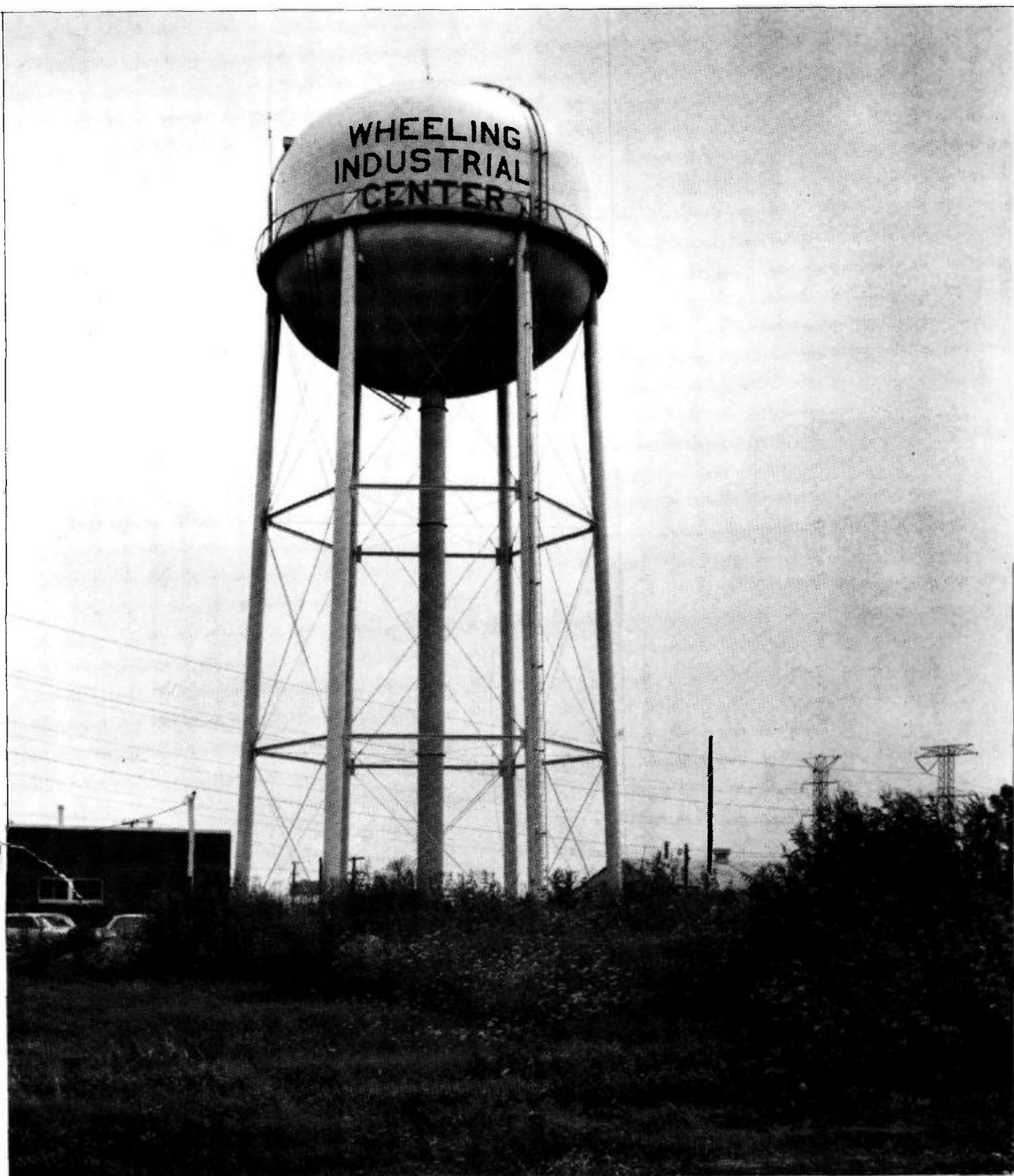
One of Six Wells
